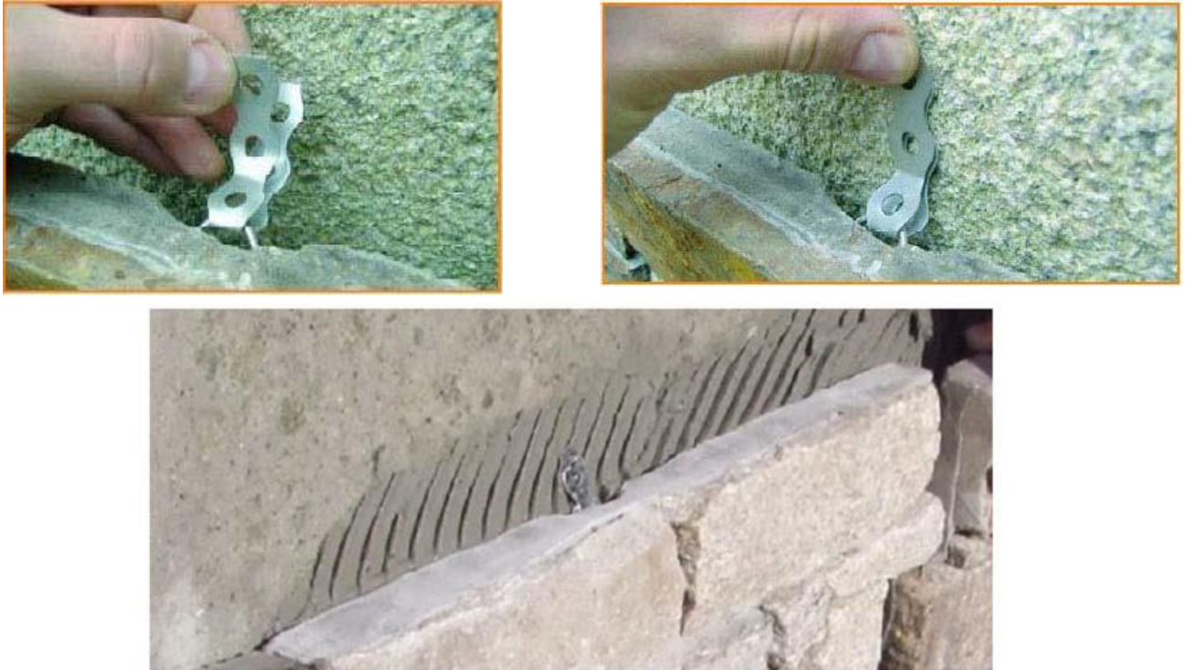
Figure 6– STONEPANEL SKY: installation of the safety element
